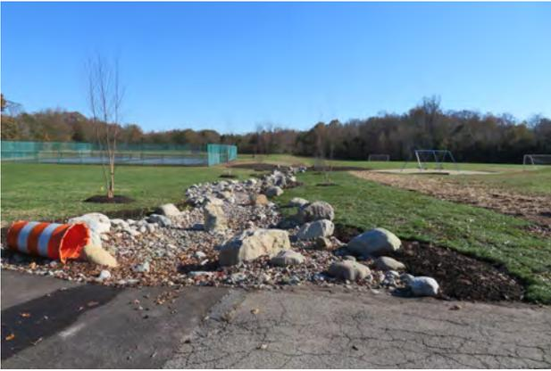
Construction is complete on the stormwater control portion of an outdoor classroom at Craik Elementary in Pomfret that will support environmental education instruction. PTRC received a Chesapeake Bay Trust Outreach and Restoration Grant to construct a stabilized swale with over 1000 native plants to address stormwater runoff into the Port Tobacco Creek from the school's buildings and parking lots.
